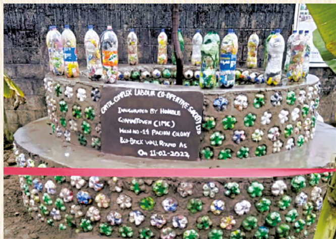
Eco-bricks bench. Arunchal Pradesh
